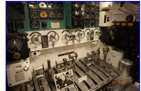
Motor Room - Propulsion Control Panel
