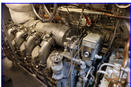
Forward Engine Room Diesel (GM278A)
